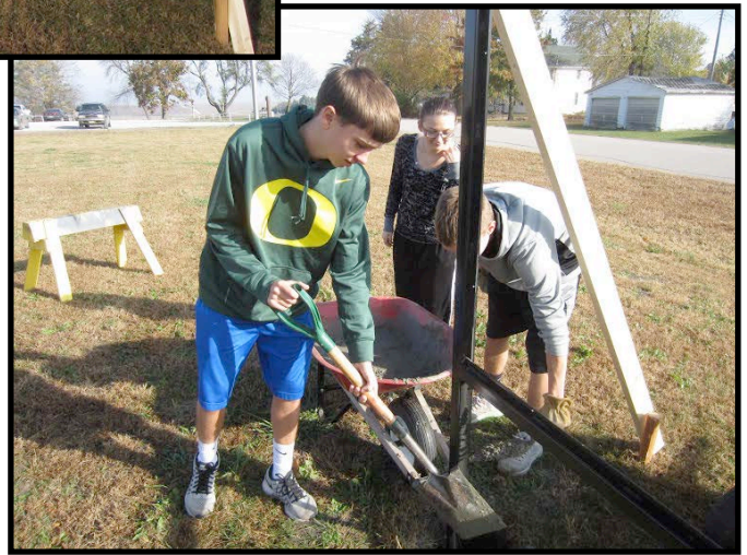
FFA Members mixed Quik Crete for the frame and back filled with rock. The sign has a front and a back message.
